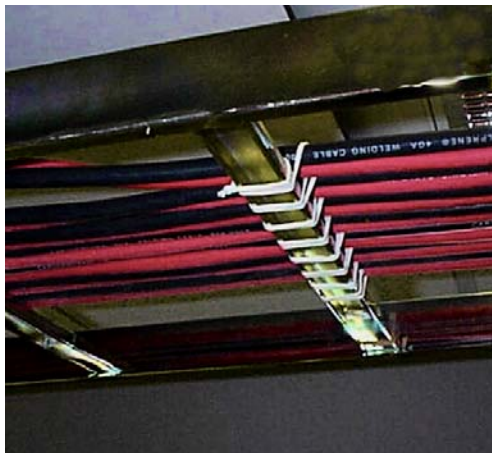
FIGURE 9-17 TELEPHONE COMPANY LACING METHODS
