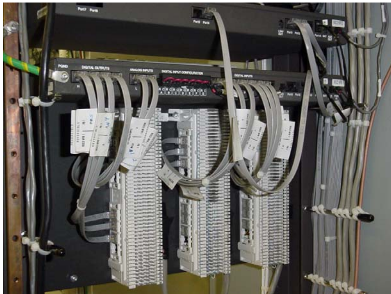
FIGURE 9-19 EXAMPLE OF CABLE LABELING
